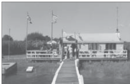
The Remsen bay house was adopted by Rich Muldowney and others in 1992 after the nor'easter.
