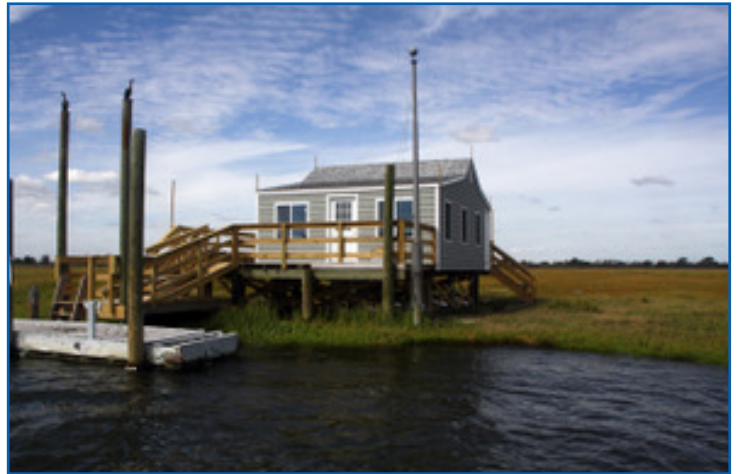
Muller bay house restored after Sandy.
